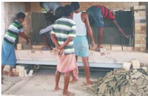
Work in progress at the clay tiles cluster
