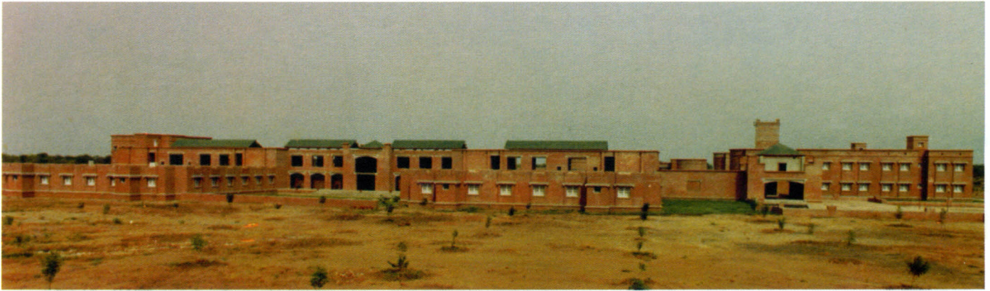
EDI campus under construction - 1984-85
