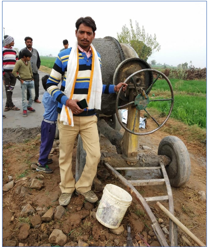
Suresh Jatav at a Construction site in his village
